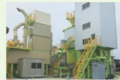
A plaster-based solidification material manufacturing facility It manufactures gypsum hemihydrate by drying gypsum powder. The facility manufactures solidification material by blending with cement and lime.
