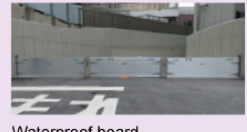
Waterproof board Waterproof boards, which are effective against water damage (internal flooding) caused by global warming
