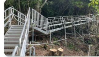
Temporary construction equipment (Other Business)
