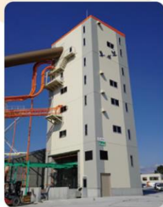
Concrete plant (BP-Related Business)
