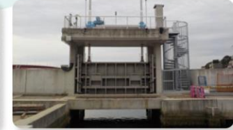
Floodgate (Other Business)
