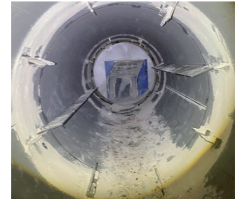
Photo 3-2: Inside of Cooling Kiln
