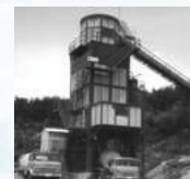
Development of u-type concrete plants (1977)
