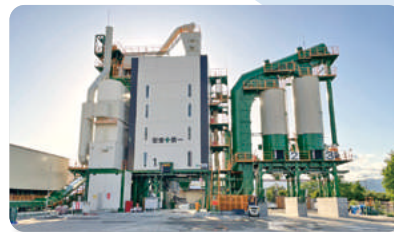
Asphalt plant (AP-Related Business)
