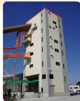
Concrete plant (BP-Related Business)
