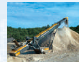
Started handling the mobile conveyor Trackstack (2018)
