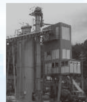
Development of compact concrete plants (1979)
